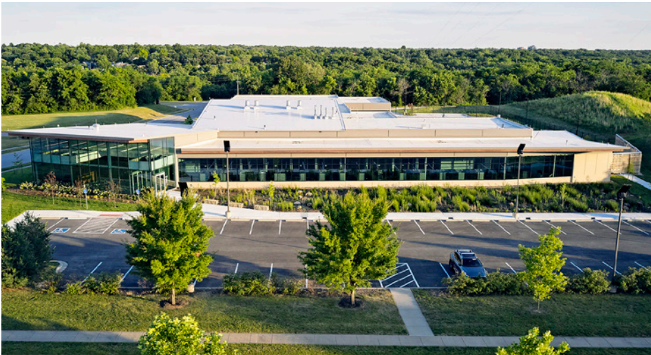
Image provided by McCarthy Building Companies
